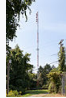
WWVU-FM antenna, Morgantown, West Virginia, 2015
